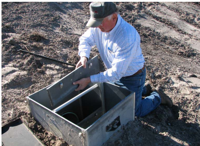
Jim installing boards in the AgriDrain water control structure. This structure allows the landowner to divert water into adjoining hay meadow.
