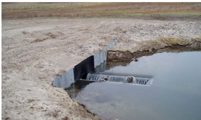
5-foot tube with weir inlet structure installed on Birdwood Creek.
