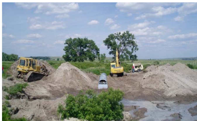
One of two ponds being constructed on Pass Creek
